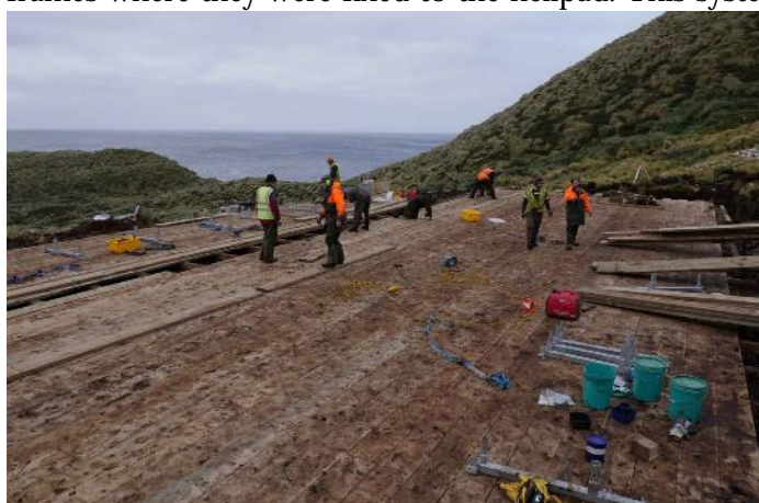
Figure 16: Helipad under construction
